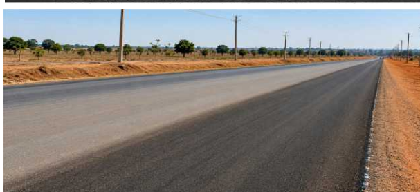
REHABILITATION OF TEGINA - KONTAGORA ROAD SECTION II, NIGER STATE
